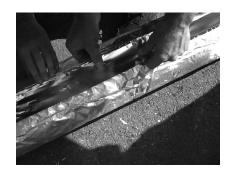
Pull back the edge of the overlap and spray additional adhesive on the inner surface of the overlapping blanket, about three feet at a time. Press the overlap together and hold for a few seconds. Once the entire seam is sealed, turn the liner over so its weight rests on the seam. Move on to measuring and wrapping the next liner section while the adhesive sets.
