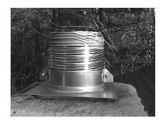
To finish your Super-Flow™ liner installation return to the top of the chimney and install the termination components. Properly installed these will both secure and stabilize the liner, and provide a weathertight assembly that prevents the entry of moisture into the flue or space around the liner.
