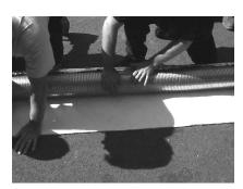
The next step is to wrap the assembled Super-Flow™ liner with Cera-Foil insulation and cover the insulation with protective SUPER SKIN stainless steel mesh. To do these steps you will want a clean, dry, relatively flat open area.
