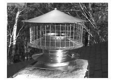
Installation of the Super-Flow™ liner is complete!
