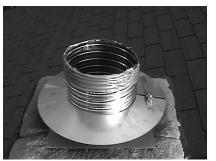
Clean the top of the projecting flue tile or the masonry crown, removing any foreign material, mortar droppings or loose granules. Make the surface relatively smooth and fill any significant cracks.
