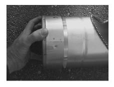
when the tee is in place. The tee holds the inner wall securely so it can be drilled without pushing the inner wall in and preventing a drill hole from being made through both walls of the two ply liner.
