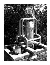
hand into flue, until base of liner TEE rests on BASE SUPPORT of flue. **NOTE:** If liner stops, lift liner 6" and drop. Repeat this a few times until liner continues down or rotate liner 360°, if possible, as this will spin SUPER FLEX tm liner off of obstruction or ledge. Center and align TEE opening if necessary.
