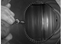
Complete installation of the tee by slipping a short section of insulation around the tee bull. It is not necessary to apply spray adhesive or SUPER SKIN, but do tape the seam with aluminum tape.
